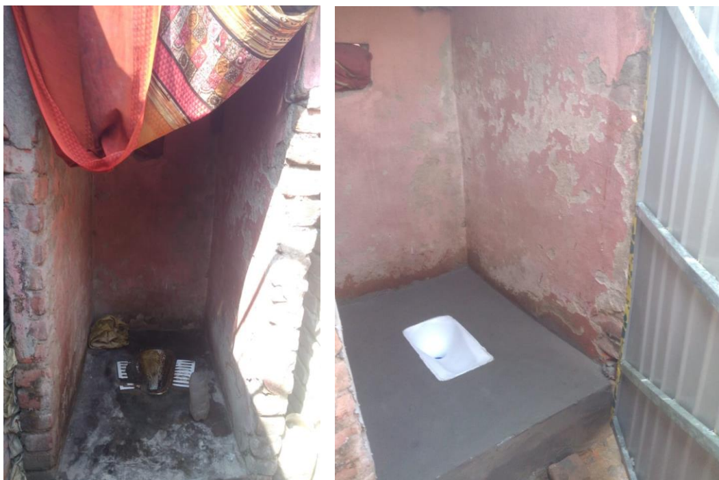
Figure 5: Pre and Post Photo after Retrofitting in Bihar
