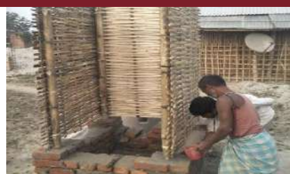
Low Cost and Sustainable constructed Toilets under FINISH Program with bamboo
