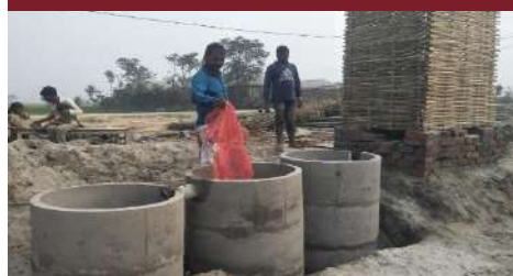
Low Cost and Sustainable constructed Toilets under FINISH Program with bamboo
